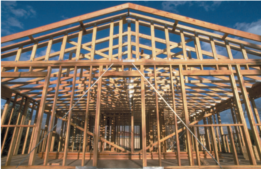
The wood frame of a new house being erected in Lone Pine, California.
