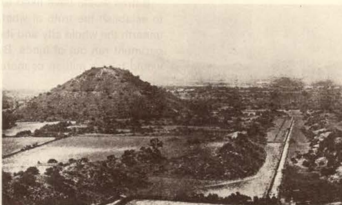
The Way of the Dead and the north and east sides of the Sun Pyramid before Batres began his excavations.
