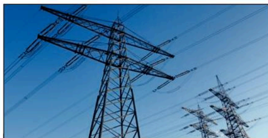
Figure 9.1.1 Overhead power lines are made of metals that are good conductors of electricity.
