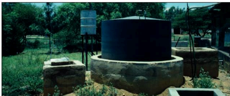
Figure 13.1.3 Biogas digesters turn animal and plant waste into methane gas.
