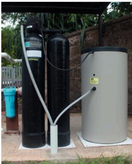
▲ Figure 21.2.2 An ion-exchange water softener. The black cylinders contain the ion-exchange resin and the grey tank contains the sodium chloride used during regeneration.
