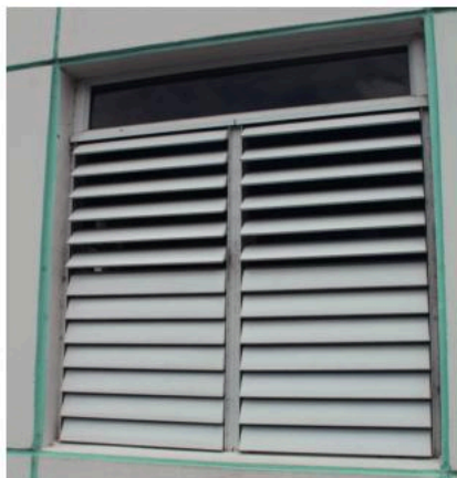
▲ Figure 18.3.1 Aluminium is used to make louvred windows
