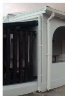
▲ Figure 16.1.4 Polyvinyl chloride is used to make guttering
