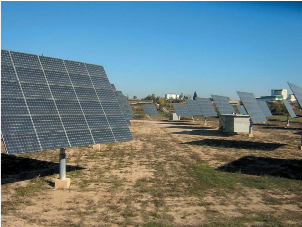
Figure 13.11 A solar farm near Lerida, Spain, which uses a pole mount with dual-axis trackers. Source: Chixoy, Wikimedia Commons.
