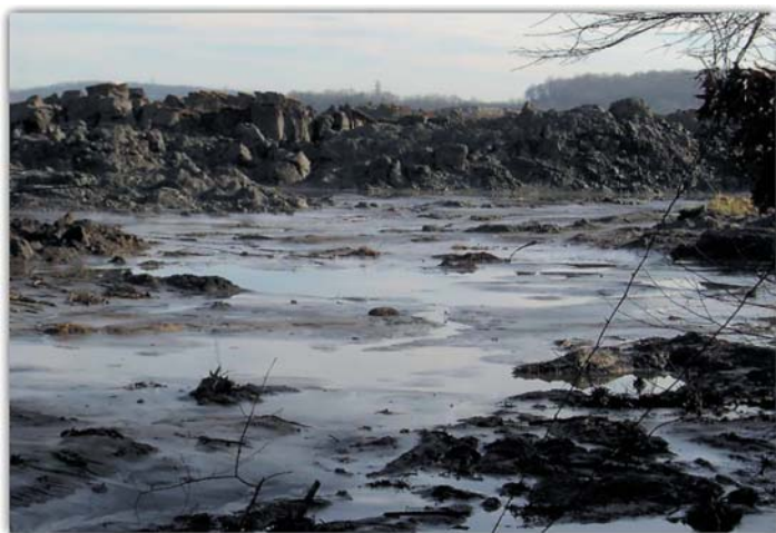
Figure 8.20 A 25-ft wall of fly ash slurry located approximately 1 mile from the original impoundment at the Kingston Fossil Plant. Source: Brian Stansberry, Wikimedia Commons.
