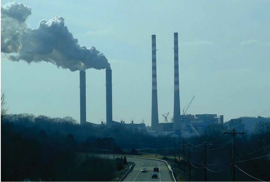
Figure 2.12 An example of tall industrial smoke stacks used to release pollutant emissions above the thermal boundary layer. Source: Steven Greenwood, Wikimedia Commons.
