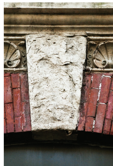
Figure 21.20 A “before and after” image showing the effects of acid rain on decorative building details.
