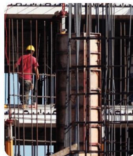
▲ Iron rods give the building strength.
