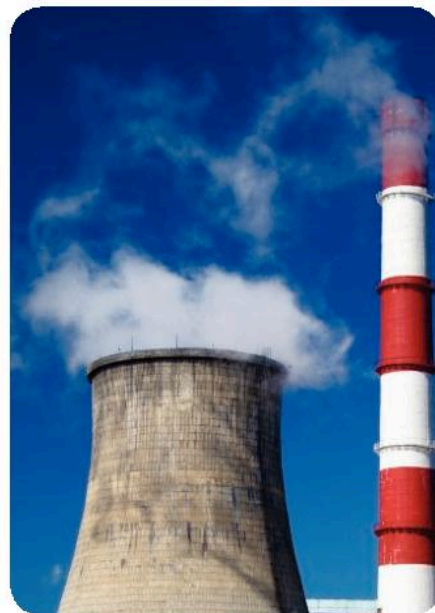
▲ Flue gas desulfurisation removes sulfur dioxide from waste gases.
