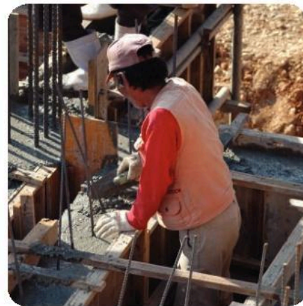
▲ Cement: limestone heated with clay, and gypsum added to slow down the 'setting' process.
