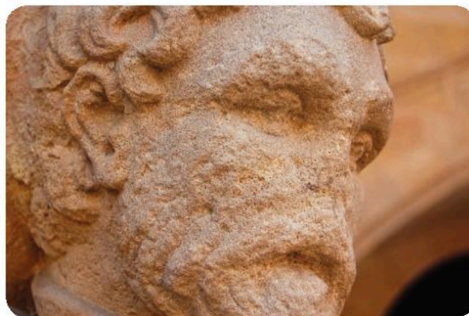
▲ The effect of acid rain on a limestone statue.
