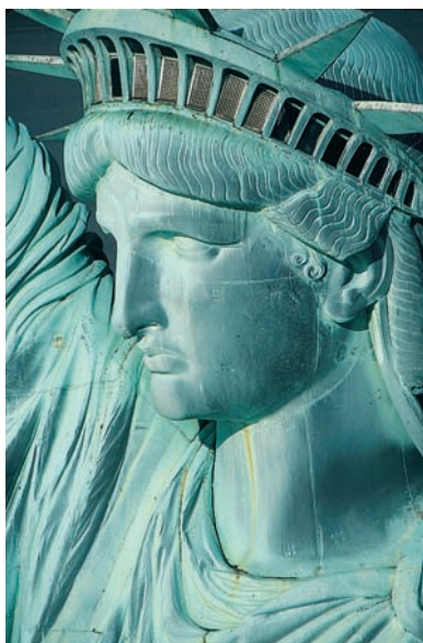
Figure 1.3 The green color of the Statue of Liberty results from the reaction of the copper skin of the statue with the components of air. That copper will react with the components of air is a chemical property of copper.
