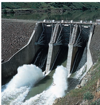
Figure 7.1 The water in the lake behind the dam has potential energy as a result of its position. When the water flows over the dam, its potential energy becomes kinetic energy that can be used to turn the turbines of a hydroelectric plant.
