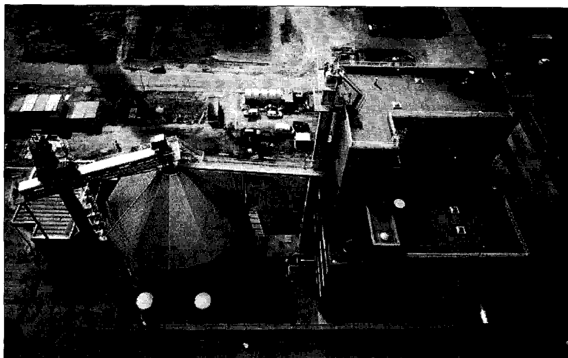
Figure 10.47 The AMER gasification plant in the Netherlands.
