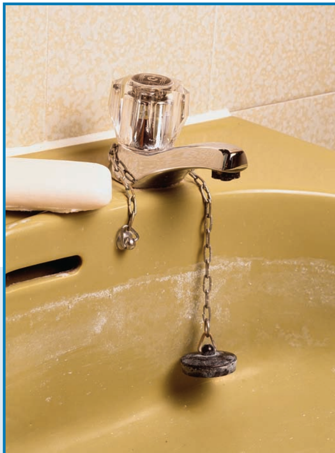
Figure 5.3 As seen on the side of the tub and drain stopper ( right ), a white residue known as soap scum forms when soap reacts with calcium salts present in hard water.
