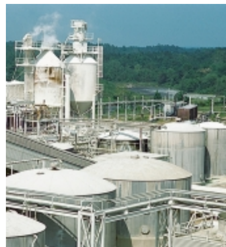
▲ The manufacture of cement begins with the thermal decomposition of limestone, \text{CaCO}_3 , in large kilns.
