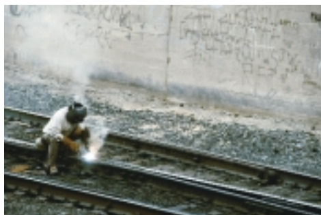
▲ FIGURE 8.7 The thermite reaction of aluminum with iron(III) oxide is so strongly exothermic and releases so much heat to the surroundings that the products become molten.
