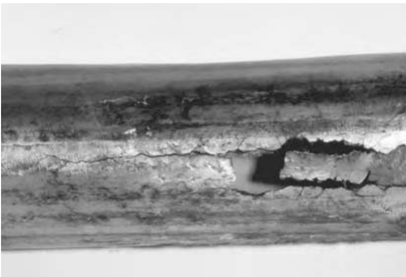
Fig. 5 External SCC of a stainless steel pipe after contact with wet, chloride-containing, thermal insulation.
