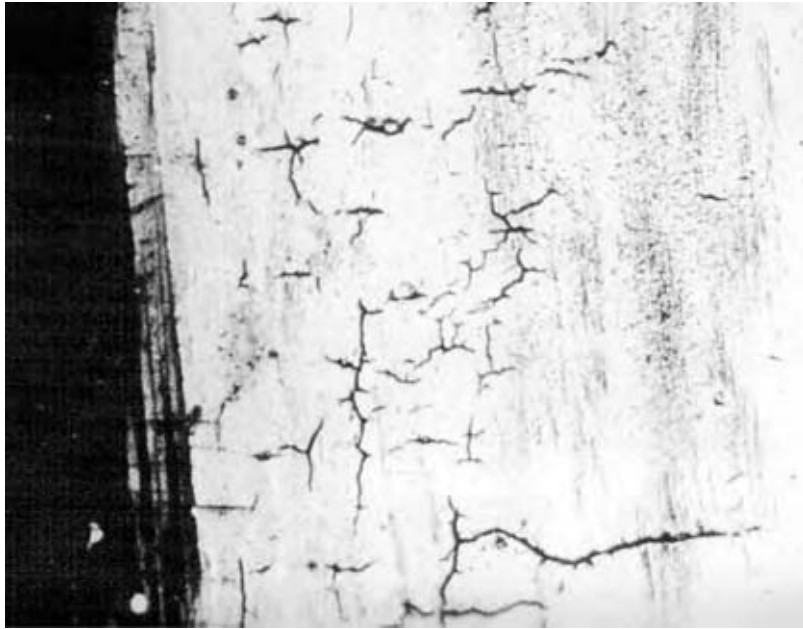
Fig. 6 Environmentally assisted cracking of a weld in a deaerator, caused by a combination of static residual and cyclic operating stresses, and revealed by magnetic particle inspection.
