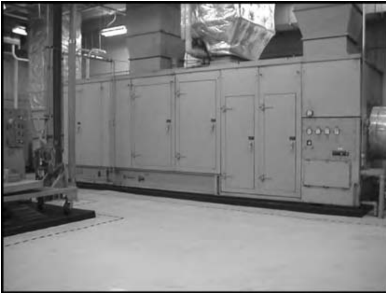
Fig. 12 Centaur H turbine installation. (View this art in color at www.dekker.com .)
