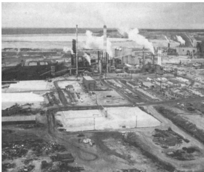
Fig. 2. General view of upgrading plant for processing bitumen mined from Athabasca deposit. In the foreground is the sulfur stockpile; in the background is a tailings pond. Right background shows the extraction plant; left is the coke pile. (Alberta Government Photographic Service)
