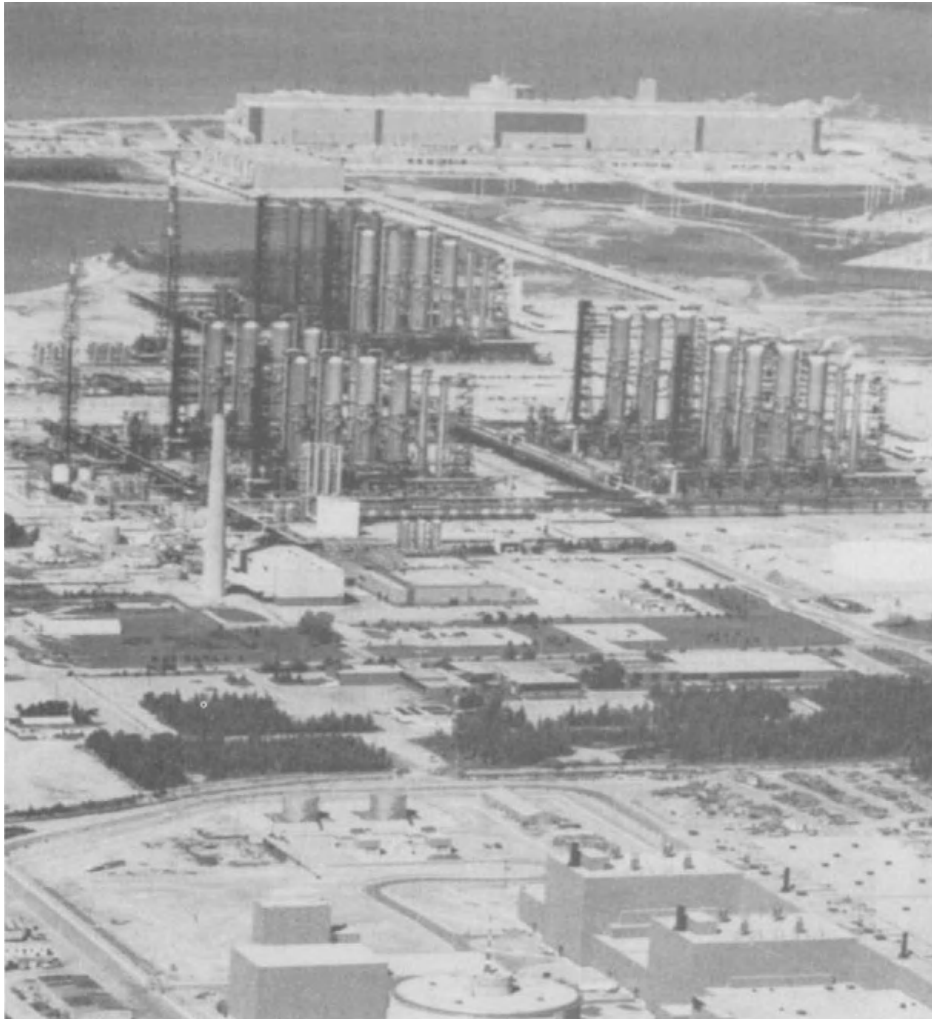
Fig. 25. Series of towers comprising part of the heavy water production plant at Ontario Hydro's Bruce nuclear power complex near Tiverton on the shores of Lake Huron. Heavy water is a clear, colorless liquid that looks and tastes like ordinary water. It occurs naturally in ordinary water in the proportion of approximately one part heavy water to 7000 parts of ordinary water. While ordinary water is a combination of hydrogen and oxygen ( H_2O ), heavy water ( D_2O ) is made of up of deuterium—a form, or isotope, of hydrogen—and oxygen. Deuterium is heavier than hydrogen in that it has an extra neutron in its atomic nucleus, so heavy water weighs about 10% more than ordinary water. It also has different freezing and boiling points. It is the extra neutron that makes heavy water more suitable than ordinary water for use in CANDU nuclear reactors as both a moderator and a heat transport medium. (Ontario Hydro, Toronto, Ontario, Canada)
