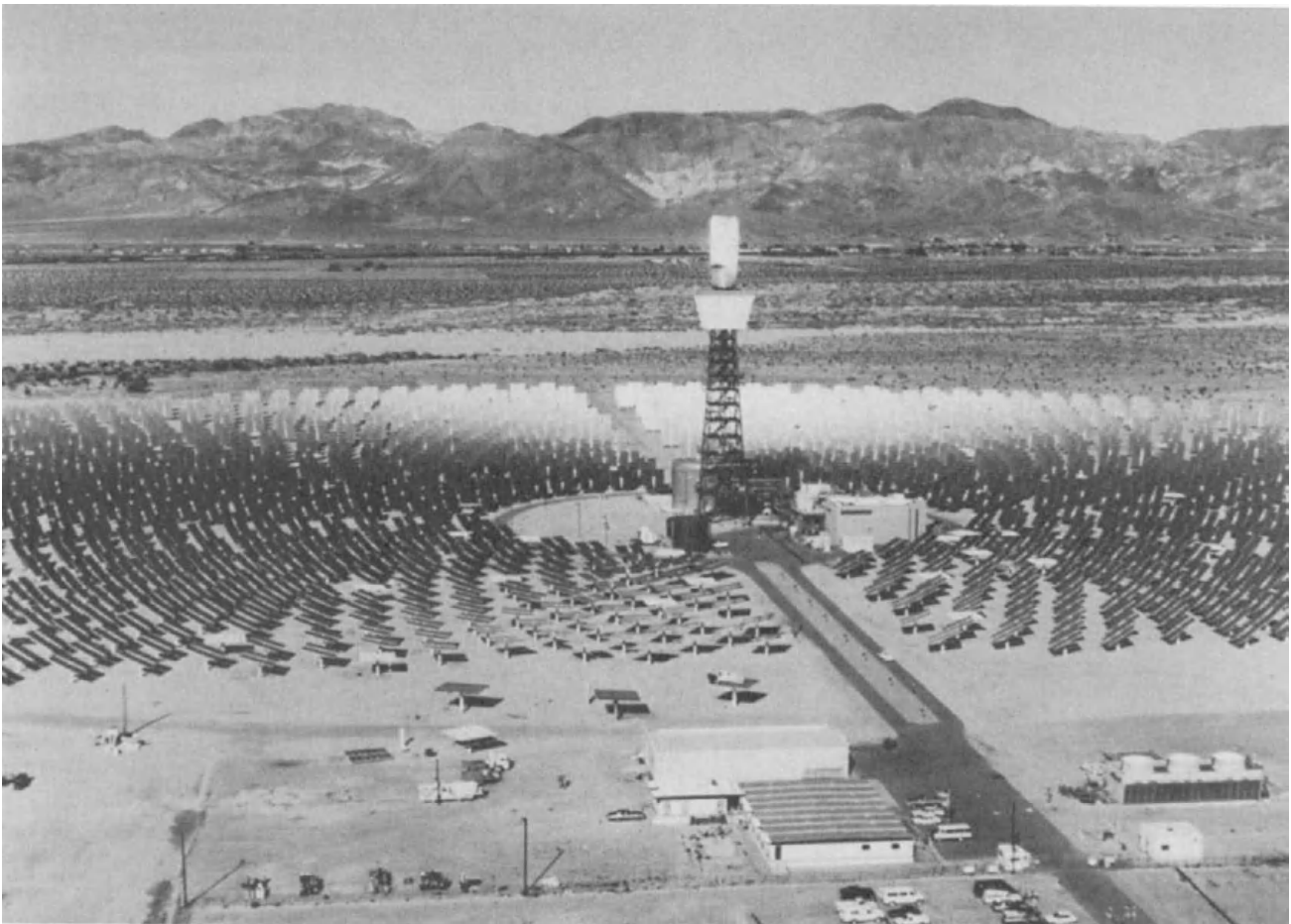
Fig. 16. Panoramic view of the world's largest solar thermal electric power plant, located on the Mojave Desert, near Daggett, California. The 10 megawatt (electric) facility commenced operation in 1982 and achieved design capacity in 1984. The collector tower (receiver upon which solar energy is reflected) is located atop a 300-foot (91-meter) tower. The north field of heliostats (mirrors kept in synchronism with the movement of the sun), 1240 in number, is shown in background; the south field (578 heliostats) is shown in foreground. Operating facilities, turbine generators, and storage tank are shown in circular middle section under the tower. The facility is operated by Southern California Edison and the Los Angeles Department of Water and Power, in conjunction with the U.S. Department of Energy and the California Energy Commission
