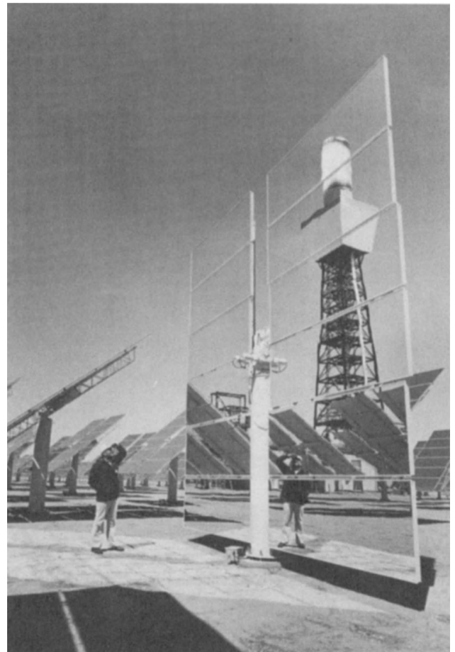
Fig. 18. Close-up of a heliostat rack assembly shown in vertical position for demonstration purposes. Note reflection of tower in mirrors. Solar One has a total of 1818 heliostats
