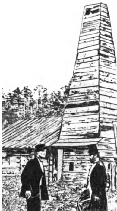
Fig. 11. Colonel Edwin Drake (right) and Peter Wilson, a druggist who endorsed a $500 bank loan for Drake, confer in front of the world's first commercial oil well near Titusville, Pennsylvania. Initially, Drake rigged a large wheel powered by steam to raise and lower a cable and iron bit. Later connected to a crude drill pipe and pump, this well produced about 35 barrels a day. (ca. 1861)
