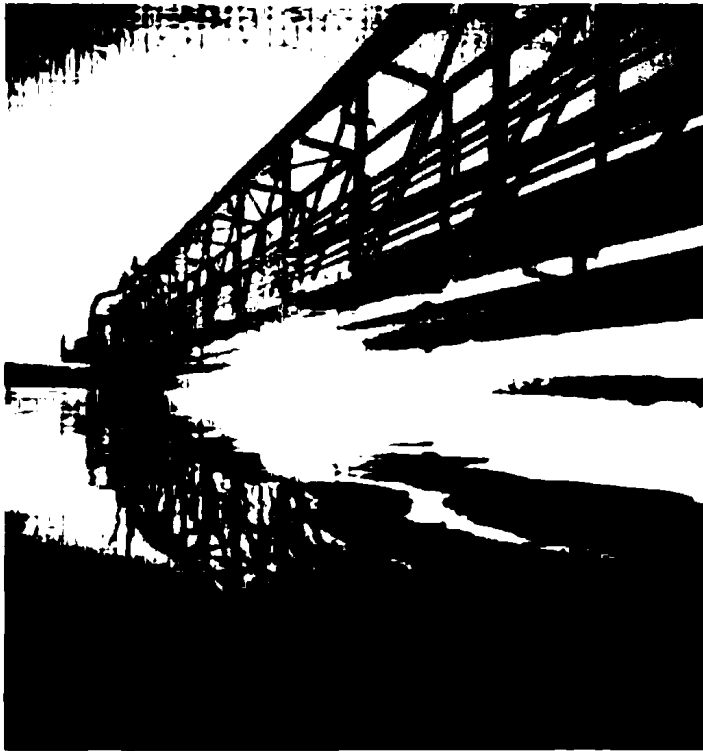
Fig. 1. Beneficiation of basic minerals involves wet operations requiring large volumes of water. Here copper tailings from a mining operation are settled in a 275-foot (84-meter) diameter thickener which handles over 2000 gallons (76 hectoliters) per minute and some 13,000 tons (11,795 metric tons) of ore per day. Underflow solids are disposed of by pumping to tailing ponds. Clarified water is returned to the mill process, thus avoiding waste of water
