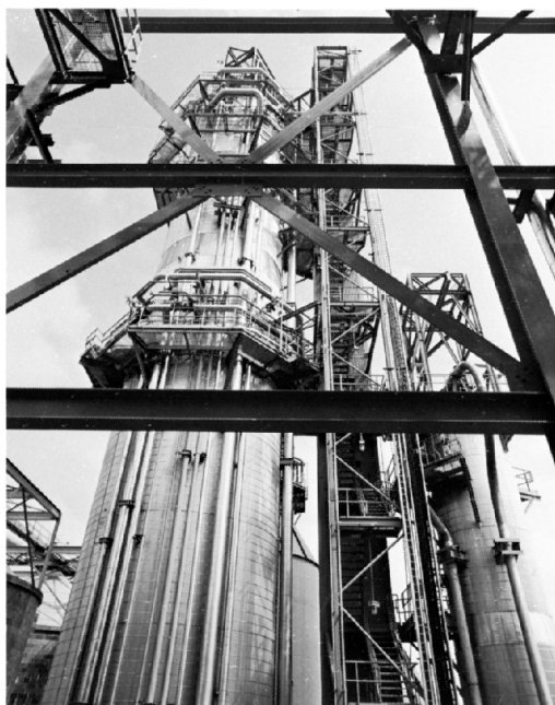
FIGURE 3 The modern Kamye continuous digester, heart of the Kraft pulp mill. [Photo courtesy of Leaf River Corp.]
