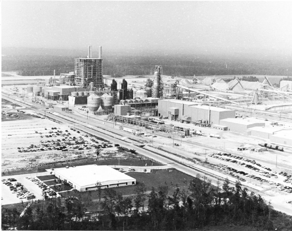
FIGURE 1 Overview of the recently completed bleached Kraft pulp mill built by Leaf River Forest Products in Mississippi. [Photo courtesy of Leaf River Corp.]
