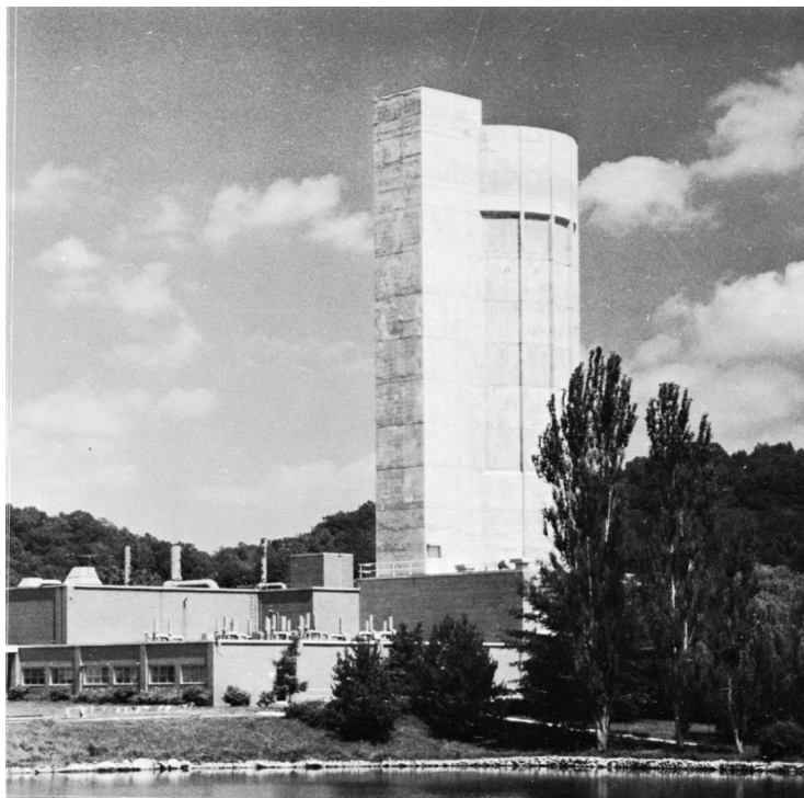
FIGURE 11 A view of Oak Ridge National Laboratory's electrostatic tandem-type heavy ion accelerator, which is insulated with SF 6 . (Courtesy of Oak Ridge National Laboratory.)
