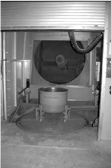
Figure 22.3.3. Wash plant for mixing vessels.
