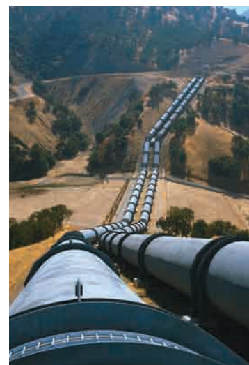
Figure 5.20 This gas pipeline harms the ecosystem by splitting up habitat.
