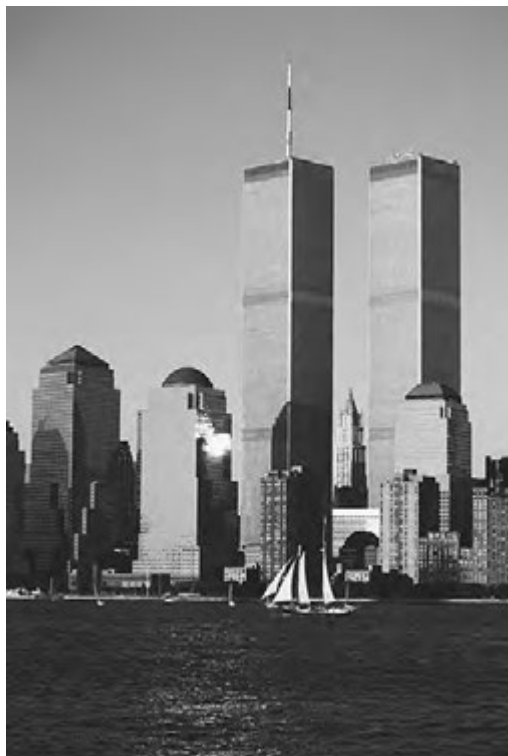
BEFORE THEY WERE DESTROYED BY TERRORIST ATTACKS ON SEPTEMBER 11, 2001, THE TWIN TOWERS OF THE WORLD TRADE CENTER IN NEW YORK CITY GLEAMED WITH A CORROSION-RESISTANT COVERING OF ALUMINUM. (Bill Ross/Corbis. Reproduced by permission.)
