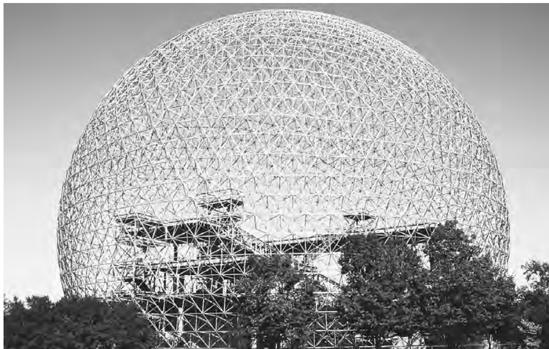
A GEODESIC DOME IN MONTREAL, QUEBEC, CANADA. SUCH DOMES ARE NAMED AFTER THEIR DESIGNER, R. BUCKMINSTER FULLER, AND EVENTUALLY PROVIDED THE NAME FOR THE CARBON MOLECULES KNOWN AS BUCKMINSTERFULLERENES. (Lee Snider/Corbis. Reproduced by permission.)
