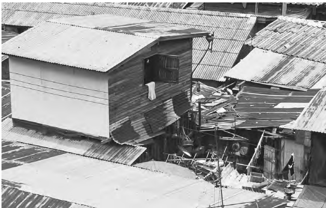
MOST “TIN” ROOFS NOW CONSIST OF AN IRON OR STEEL ROOF COVERED WITH ZINC, NOT TIN. (John Hulme; Eye Ubiquitous/Corbis. Reproduced by permission.)
