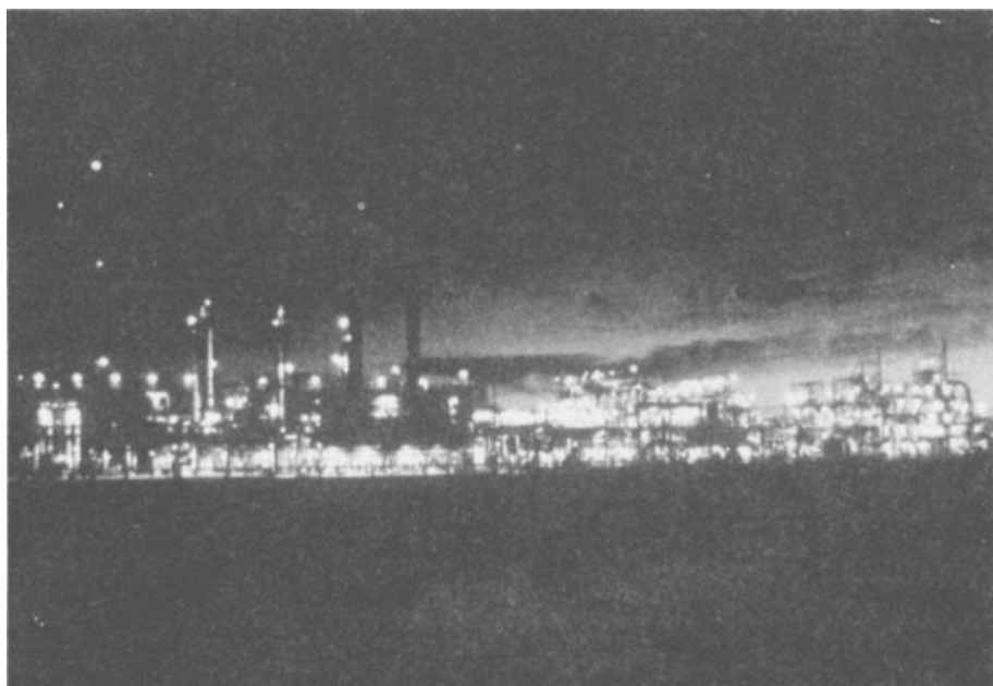
Figure 25.1 Sunset on a chemical plant. (Courtesy of BP Chemicals, Alvin, Texas)
