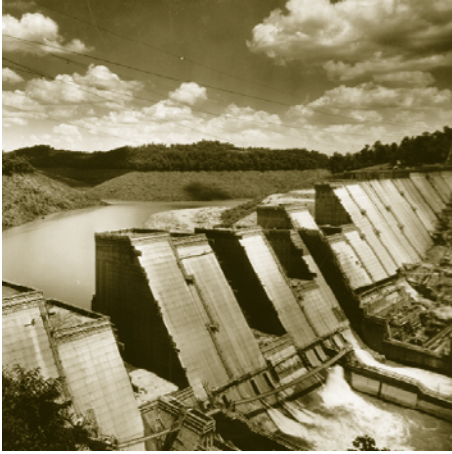
Tennessee Valley Authority (TVA) The Norris Dam on the Clinch River was built in 1933–36 as a major project of the TVA.
