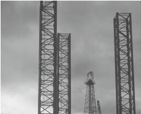
derrick Oil derrick at a California oil field. The term “derrick” was first applied to a structure used to hang criminals, from the name Thomas Derrick, a well-known London hangman.
