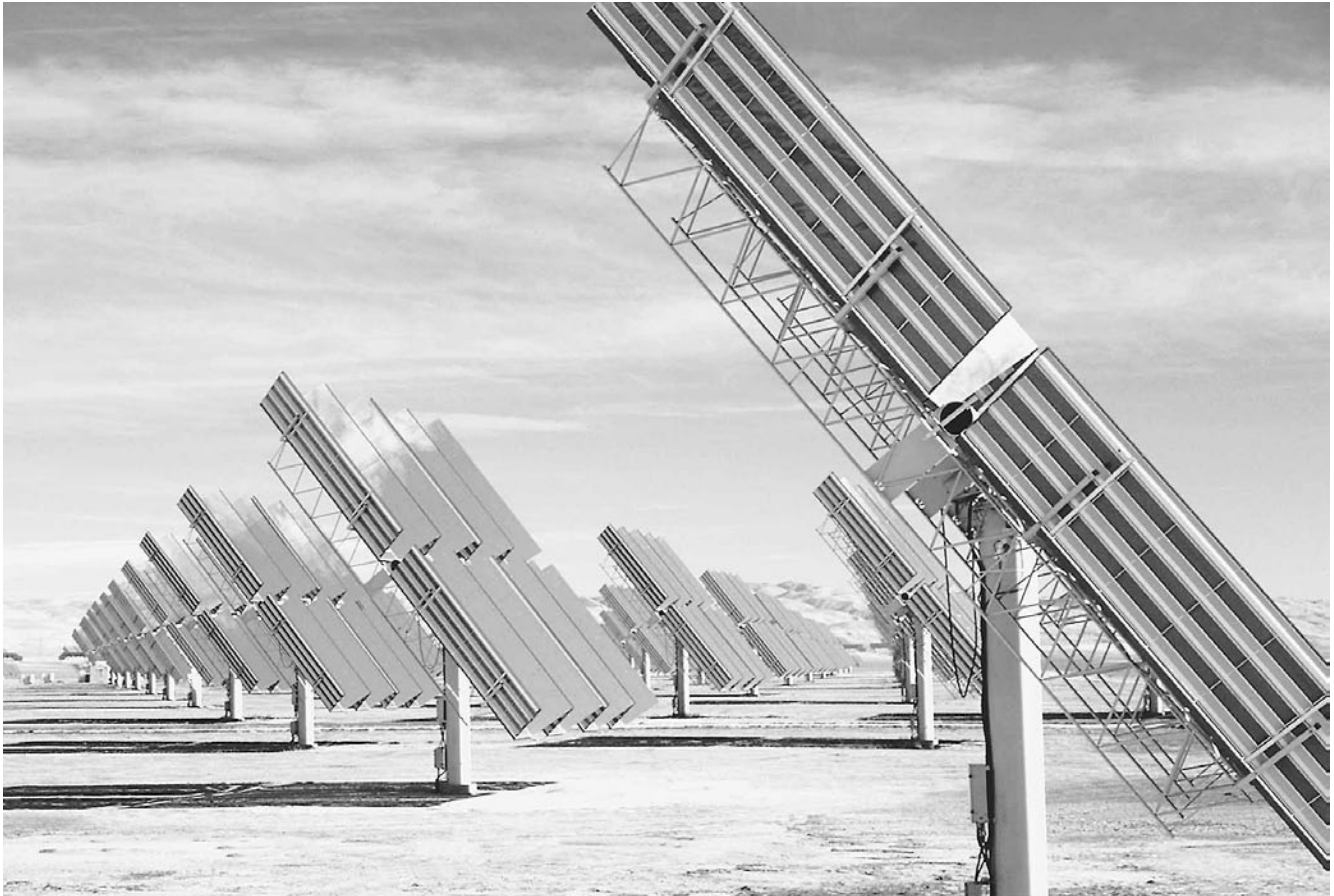
Solar collector panels. (Digital Stock)
