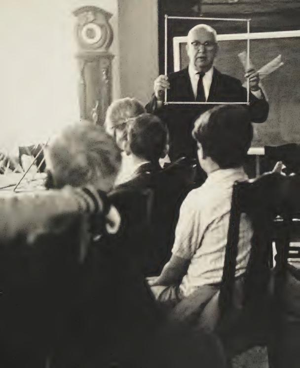
We take a side out of the square and... suddenly it's very stable. It doesn't get all flexible the way it had been with the square. So this is what we call tri-angle, three angles. And triangle, with its three angles, is the only stable structure.
