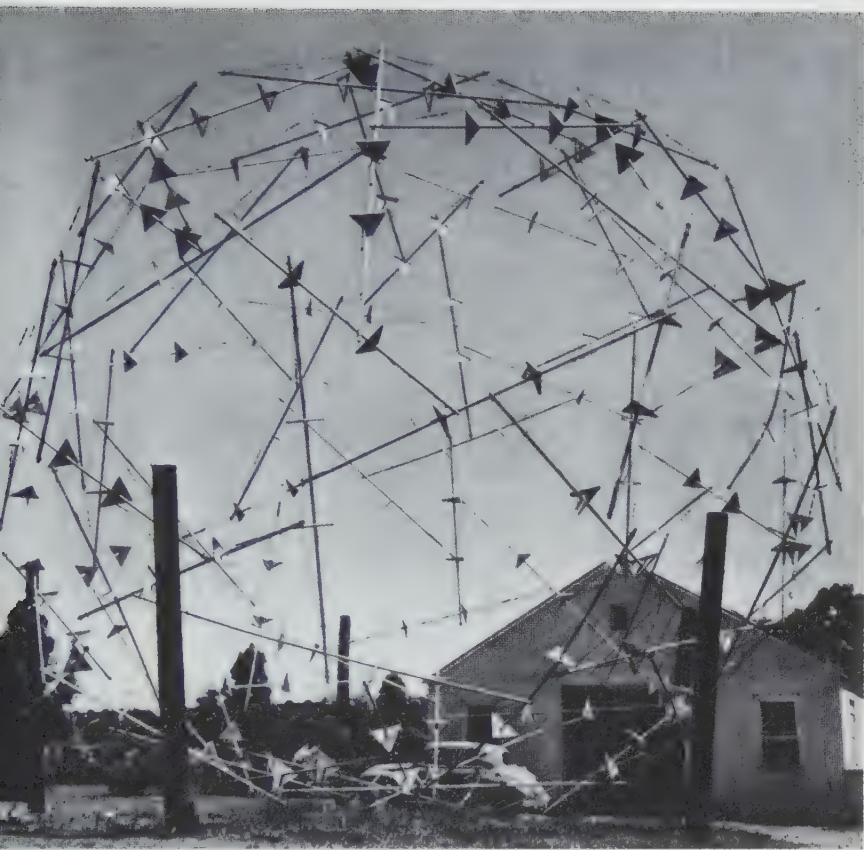
Tensegrity Sphere. The 40-foot sphere was built from 90 independent metal struts held together by a network of cables, which evenly distributed loads throughout the lightweight structure.
