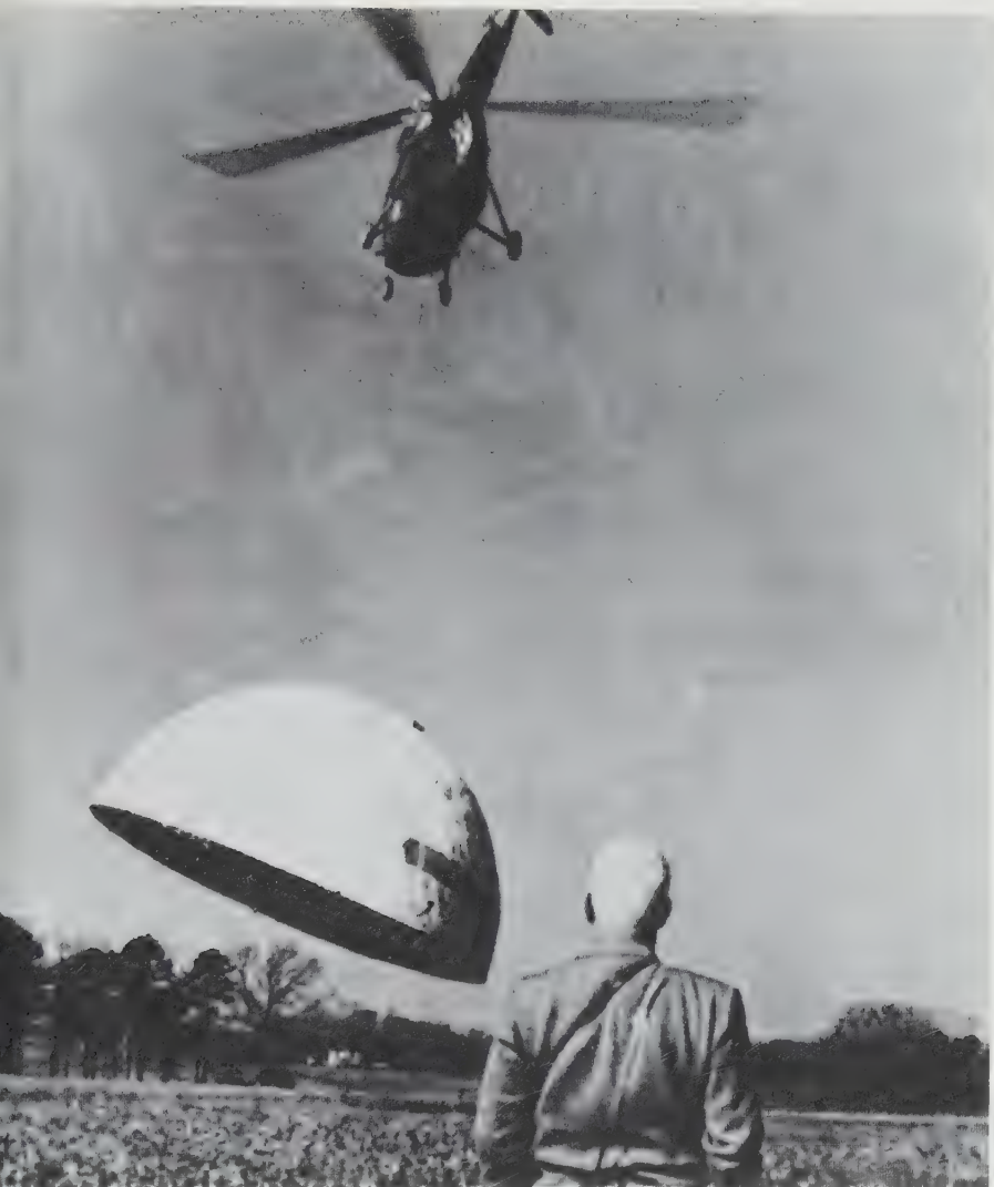
Marine Corps lifting Fuller's 30-foot wood and plastic dome at Orphan's Hill, North Carolina, 1954
