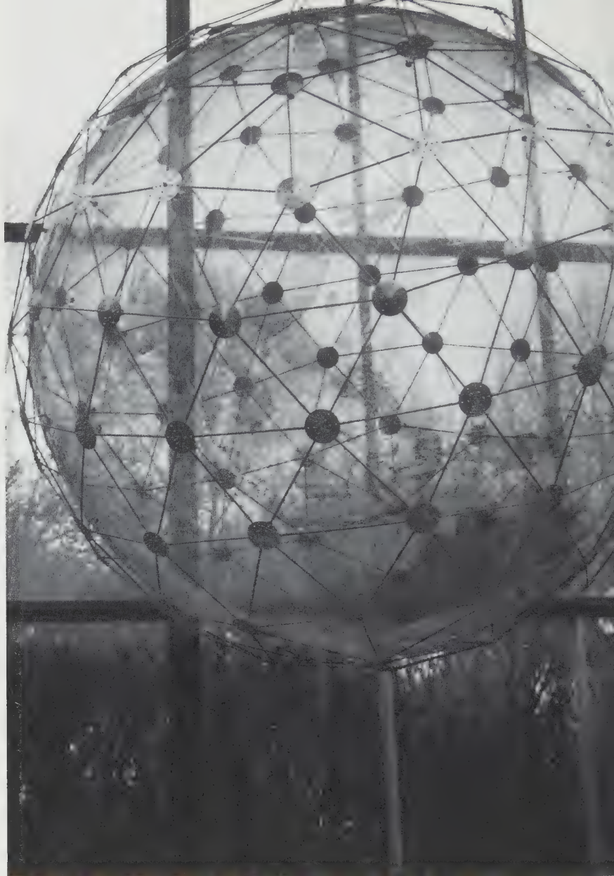
Geoscope, constructed of clear plastic inscribed with the continents and hung from a network of hollow metal tubing, about 1960
