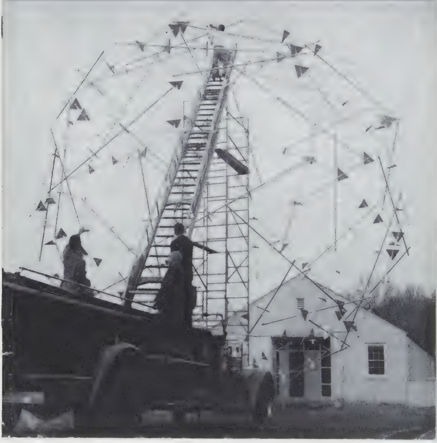
Tensegrity Sphere, built on the Princeton University campus by Fuller and students, featured in the 27 November 1953 edition of the Princeton Alumni Weekly . The cover caption reads, "With the help of the fire department apparatus, graduate students put the final touches on an architectural experiment which has excited nationwide attention."
