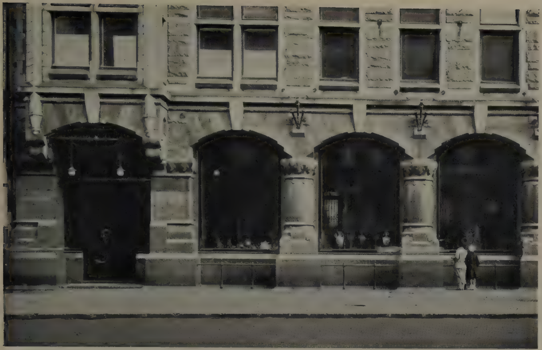
8. Fabergé's shop in Morskaya Street, St. Petersburg
