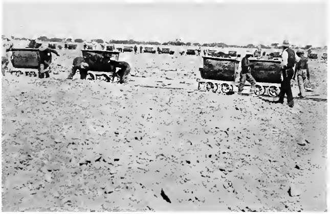
ON THE FLOORS LOADING BLUE EARTH FOR THE WASHING MACHINES, KIMBERLEY MINES
