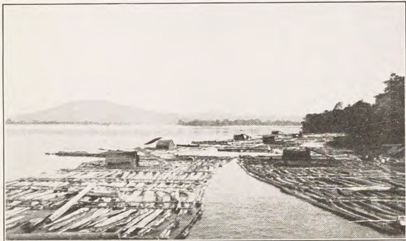
2. RAFT OF TEAK LOGS ON THE IRRAWADY RIVER
