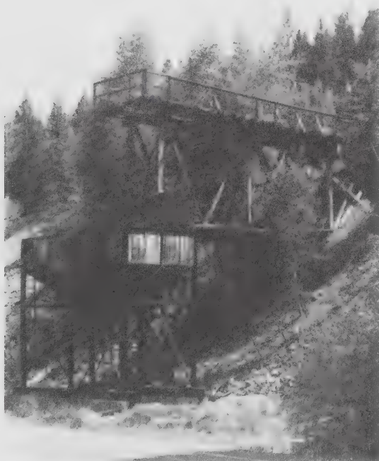
Sulfide minerals can often be found near ore-loading facilities, such as this structure near Lake City.
