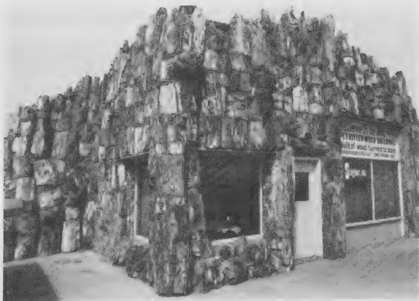
The "Petrified Service Station" in Lamar as it appears today.
