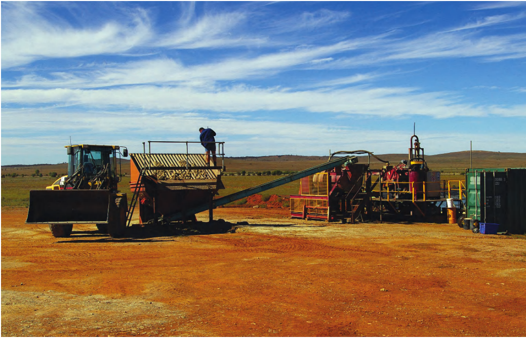
1-17: Mineral separation plant used for processing small-scale placer diamond deposits. Terowie, South Australia.
