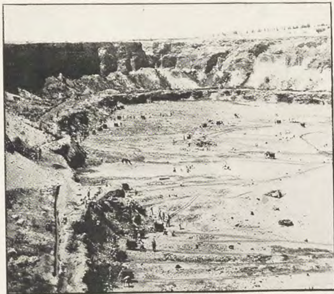
FIG. 5. WESSELTON DIAMOND MINE. OPEN WORKINGS.
