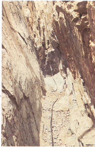
FIG. 8. Drilling prior to setting charges.
