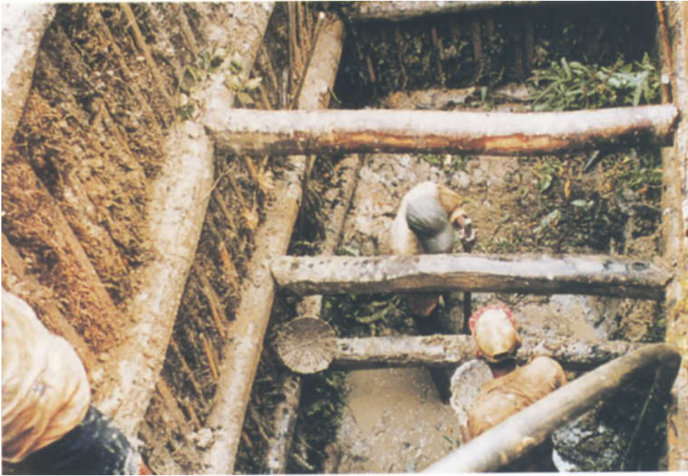
Figure 2: Typical gem pit, showing timbering and lagging of walls.
