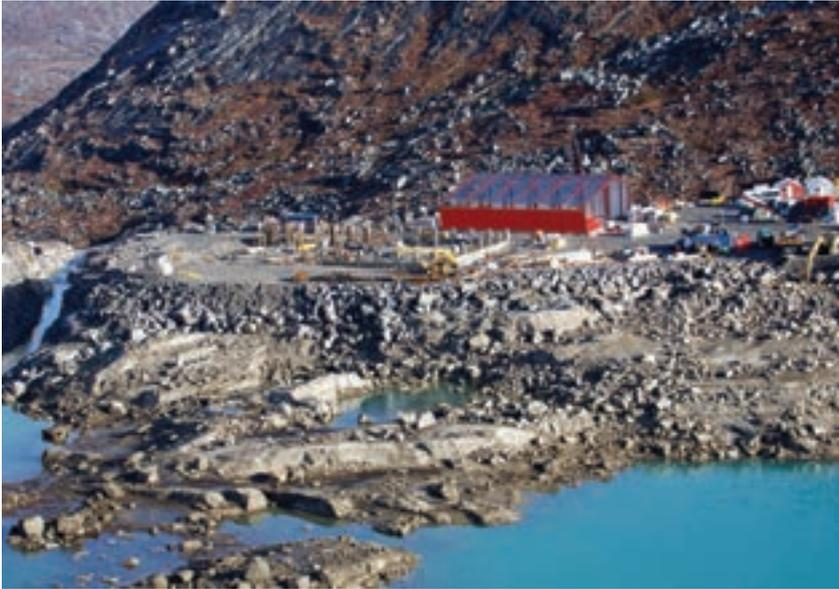
*Figure 4: This aerial photo shows the construction of the processing plant and main workshop at the Aappaluttoq deposit, well underway. The processing plant will employ dense media and magnetic separation, as well as advanced optical sorting technology to extract the corundum. Since this image was taken in October 2015, the plant building has been completed. Photo courtesy of True North Gems Inc.*
