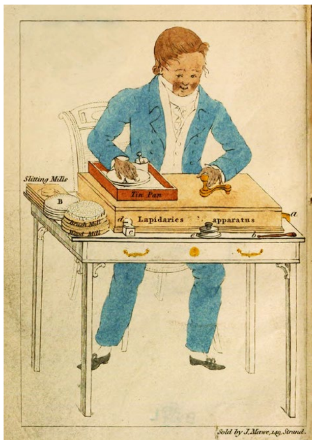
Figure 2: This illustration of a Regency-era gentleman operating a British-made portable faceting machine (Mawe 1821, facing p. 102) provides an early example of equipment designed to appeal to amateur lapidaries. It was possibly the invention of John Mawe.
