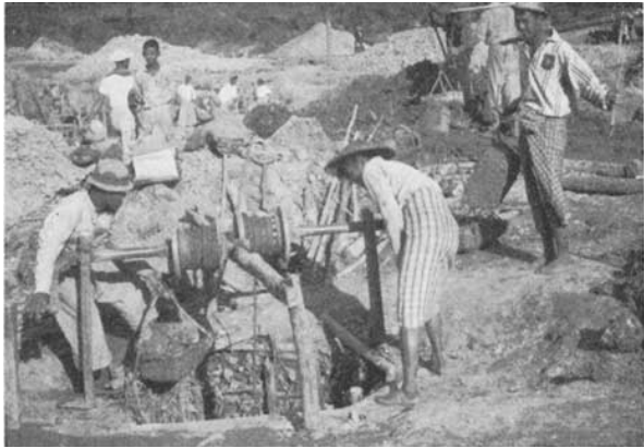
FIG. 14. The product of a deep narrow mine being winched up.
