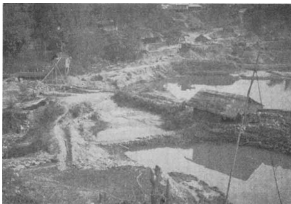
FIG. 2. Large water reservoirs in a mine field in the valley of Mogok.
