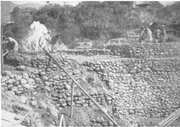
FIG. 6. View of the upper part of the so-called "machine-mine" in which a pump raises the softened "byon" or the washing water to the working level.
