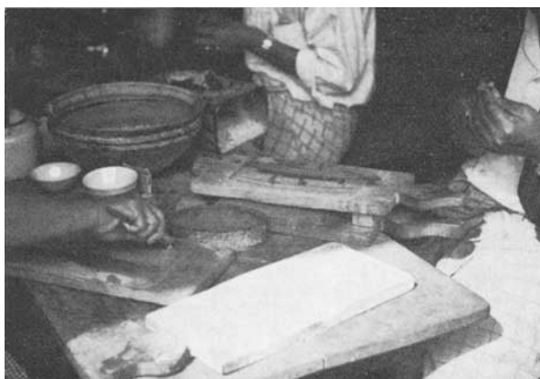
FIG. 18. Larger cabochons are worked on grinding wheels covered with carborundum.
