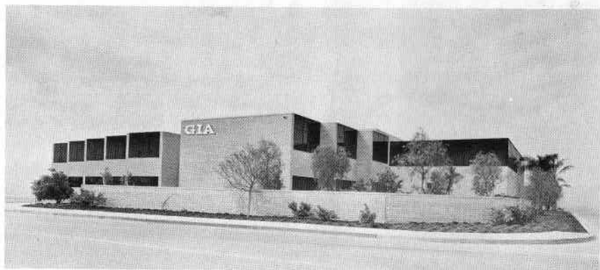
New GIA Headquarters Building, Santa Monica, California
