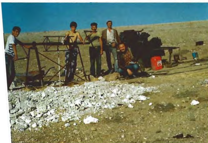
Figure 10. A "spinning wheel" (rope and pulley) system is used to remove buckets of sepiolite nodules and waste materials from one of many mining "holes" operating in the Eskisehir district.
