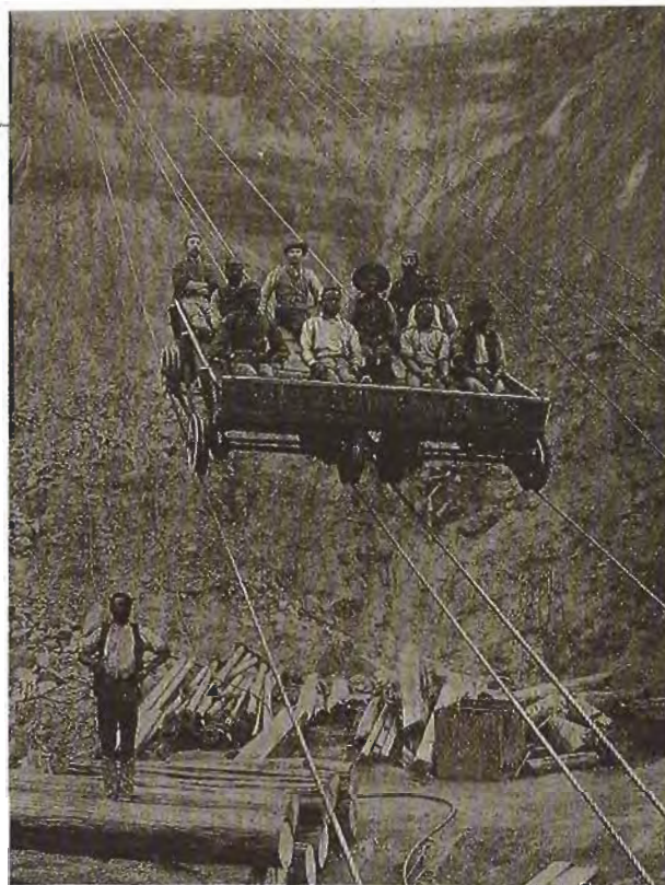
Figure 11. As the mining claims in the Kimberley area consolidated and pits got deeper, mechanization was needed to bring the miners to the ore and transport the ore to the surface. Photo from Williams, 1905.
