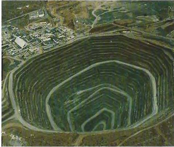
Figure 18. The Finsch mine has been a major South African diamond producer since it was opened in 1967. Mining went underground when the pit—shown here in September 1990—had reached a depth of 430 m.
