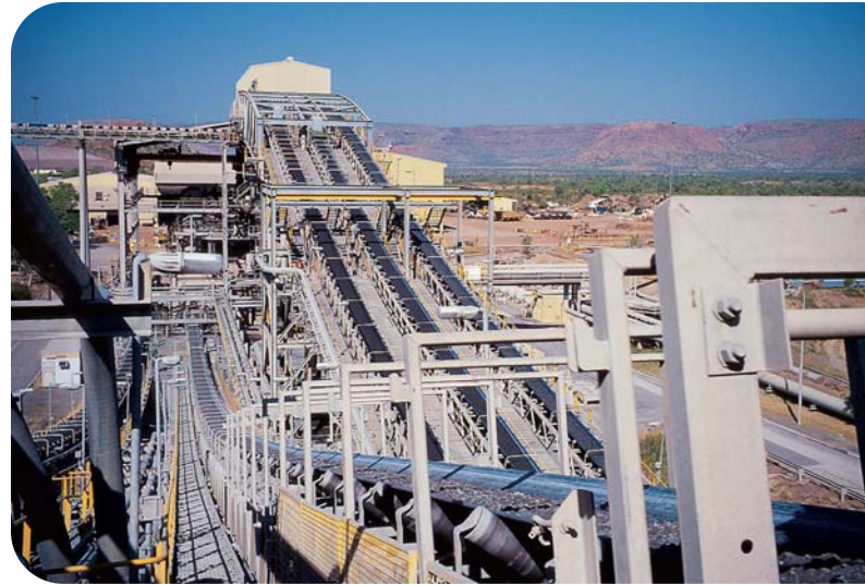
Figure 13. In a roller coaster-like operation, the crushed lamproite ore moves by conveyor belts between different stages of processing throughout the plant. Photo by James E. Shigley.
