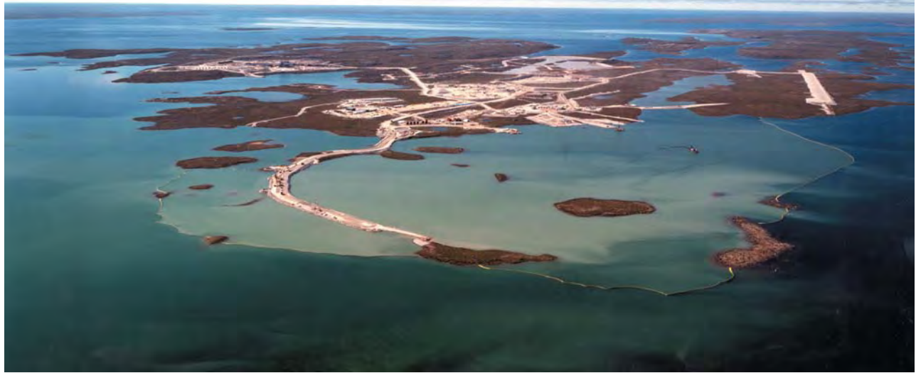
Figure 2. Construction of the Diavik mine is underway in anticipation of diamond production in early 2003. Three kimberlite pipes (A154N, A154S, and A418) are located beneath Lac de Gras in the foreground, and a fourth pipe (A21) is located under the lake on the far left of the photo. The prominent arcuate structure in the foreground is a rock dike (to be completed in fall 2001) that will be used to hold back the lake surrounding the A154N and A154S pipes to allow for open-pit mining. Silt from dike construction is carefully contained to minimize the environmental impact on the lake. The processing plant (also under construction) and camp are located in the background on the left. The disturbance in the center is a quarry that supplies rock for construction of the dike, and an airstrip is visible on the right. Photo by Jiri Hermann; courtesy of Diavik Diamond Mines Inc.
