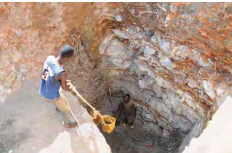
Figure 6. Ruby and sapphire mining in Winza is now concentrating more on the primary deposit located under the gem-rich soil. Mining takes place in pits that follow near-vertical amphibolite “dikes” (one is visible here between the two workers). Photo by V. Pardieu/GGL.
