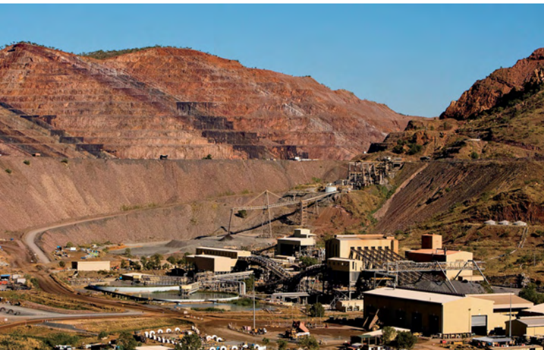
Figure 3. Australia's Argyle mine is the world's largest single diamond producer by volume. Since the 1980s, the deposit has been mined in a large open pit; the processing plant and west pit wall are shown here. Over the next few years, mining will move underground. This 2009 photo is courtesy of Rio Tinto Diamonds.
