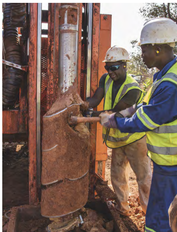
Figure 10. Workers remove the soil and gravel that come up with the auger and then dump the material into a container for further processing. Photo by Andrew Lucas/GIA.
