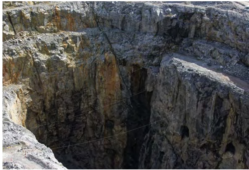
Figure 10. Kimberlite is no longer mined from either the A154 or A418 open pits—only from underground workings directly underneath. In this photo, entrances to the underground workings can be seen at several places along the pit walls. The structural integrity of the open pits is constantly monitored to ensure that the walls have not been breached by water from the lake, which would cause flooding of the underground workings. Photo by James Shigley.
