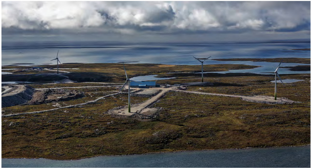
Figure 8. The wind farm, with its four large turbines, produces a significant amount of electrical power for the Diavik mine. After the rest of the facility is dismantled and removed with the end of mining, expected in 2024, the wind farm may be donated to a local community to provide electrical power. Photo courtesy of Diavik Diamond Mine.
