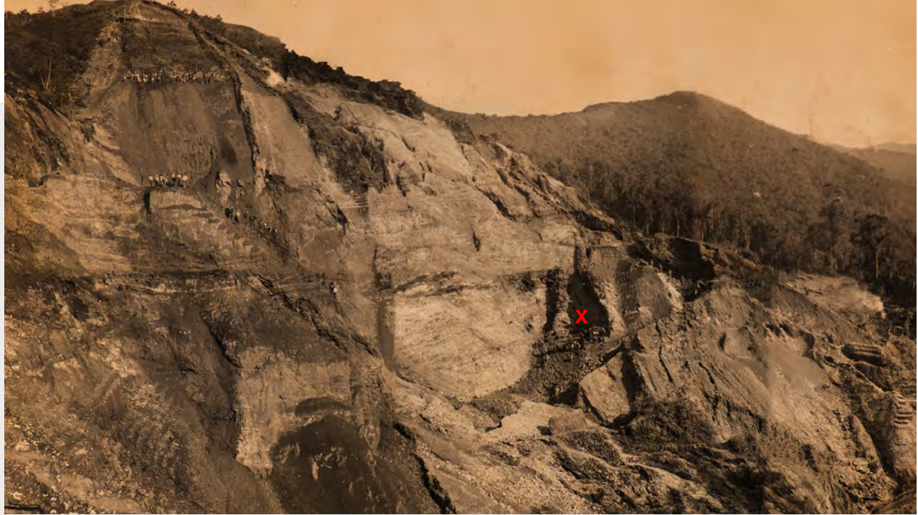
Figure B-3. This photo of the main workings at Chivor was taken by Peter Rainier in 1930. It shows the mountainside laid bare and terraced, with groups of miners using long steel rods to remove dirt, hoping to find elusive emerald veins. Once the gems were removed, a tambre was released to wash debris downhill, a technique employed by the Spanish using Chibcha aqueducts. Rainier described the location of the emerald zone, which is denoted by the red “X.” Courtesy of P.W. Rainier Jr.
