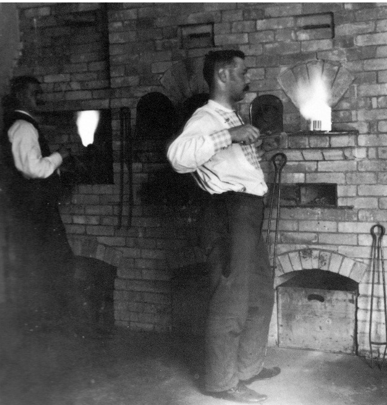
Figure 18. Fabergé's enamel firing furnace. Photo courtesy Wartski, London.
