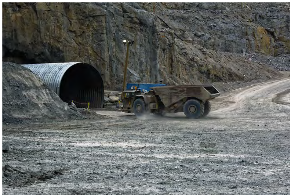
Figure 17. An ore hauler enters the access tunnel to reach the underground workings. Photo by James Shigley.
