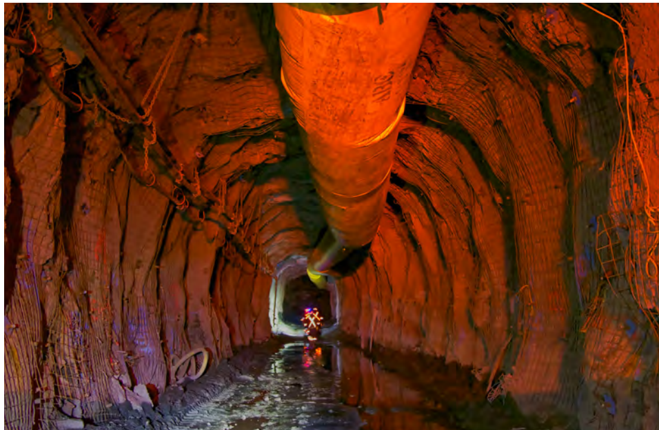
Figure 14. View of one of the underground tunnels that extend across the entire diameter of a kimberlite pipe. The tunnel's width and height must accommodate a mining vehicle. Photo by James Shigley.
