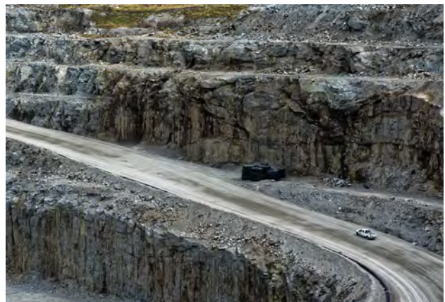
Figure 11. This view of the A418 open pit shows several of the mining benches as well as the access road that originally used to remove kimberlite ore from the pit and is now used for the underground workings. The pickup truck gives some indication of the benches' height. Photo by James Shigley.
