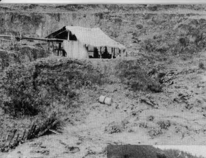
• Hut housing pumping gear in Ruby Mine.
