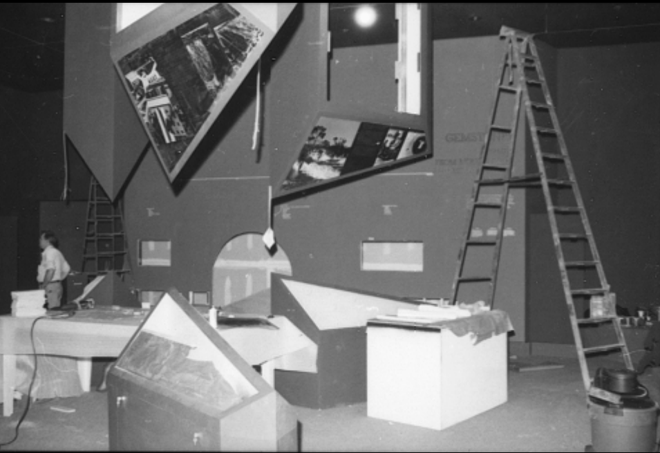
Construction of the Deutsch Gallery
