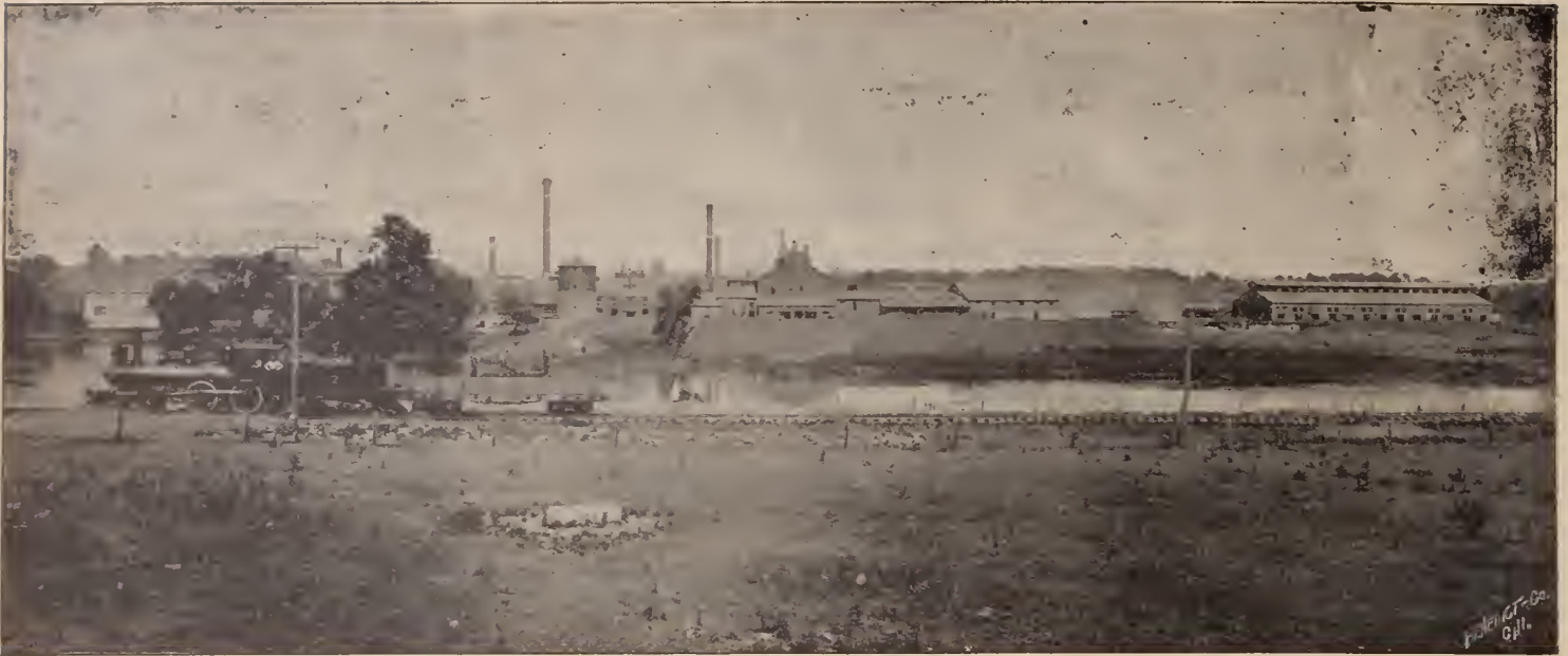
PLANT AT AURORA, ILL
