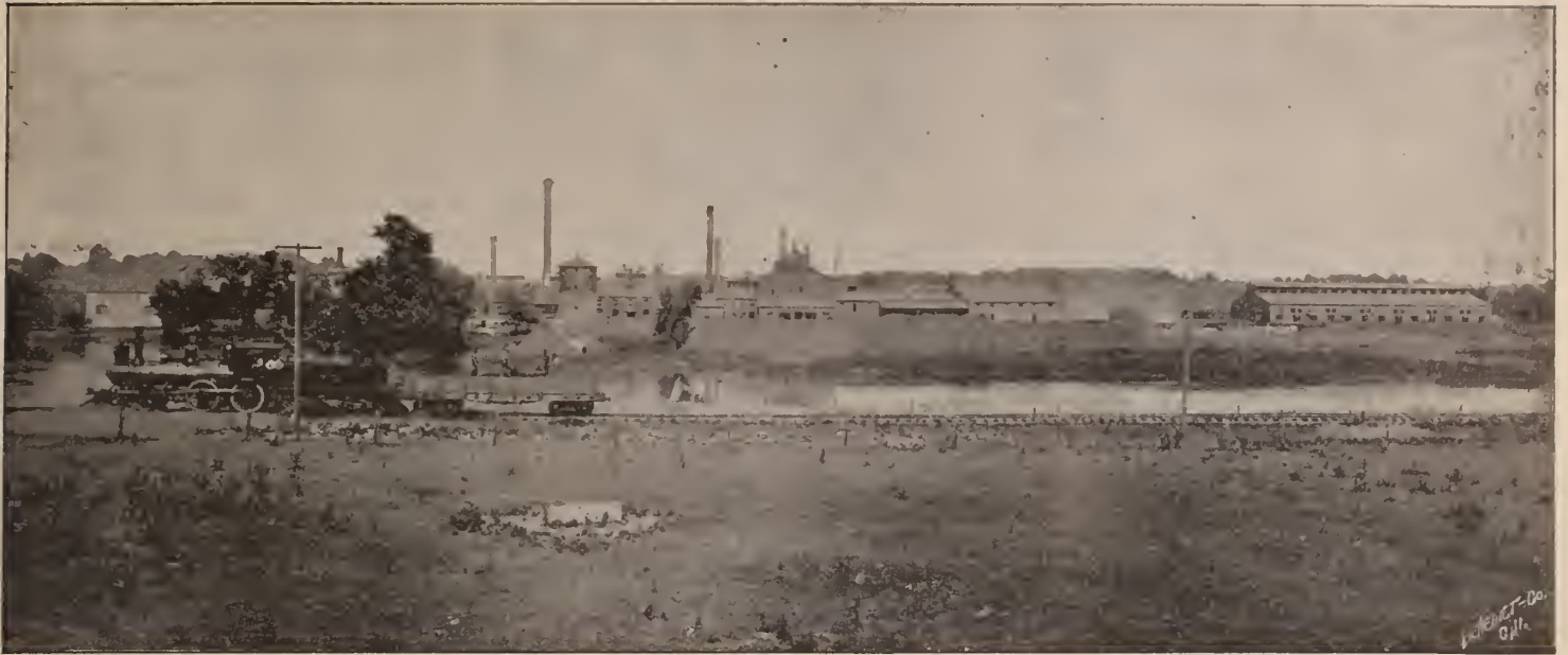
PLANT AT AURORA, ILL.
