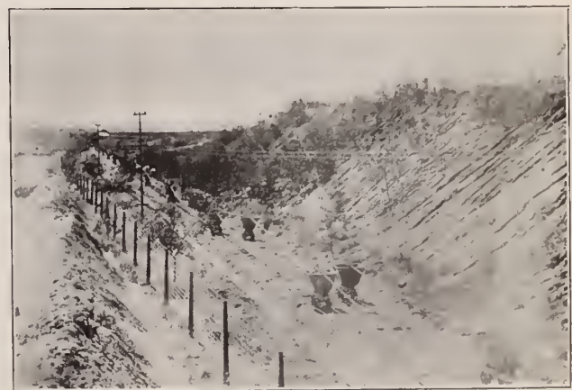
FIG. 3. CARTS HAULING BLUE GROUND TO THE FLOORS.
