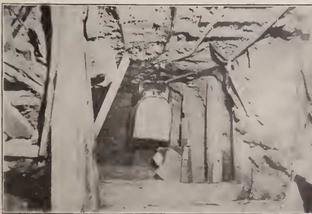
FIG. 2. TUNNEL WITH CART ACCUMULATING BLUE GROUND.
