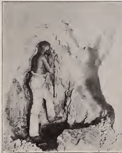
FIG. 1. MINER AT WORK DRILLING ROCK BEFORE BLASTING.
