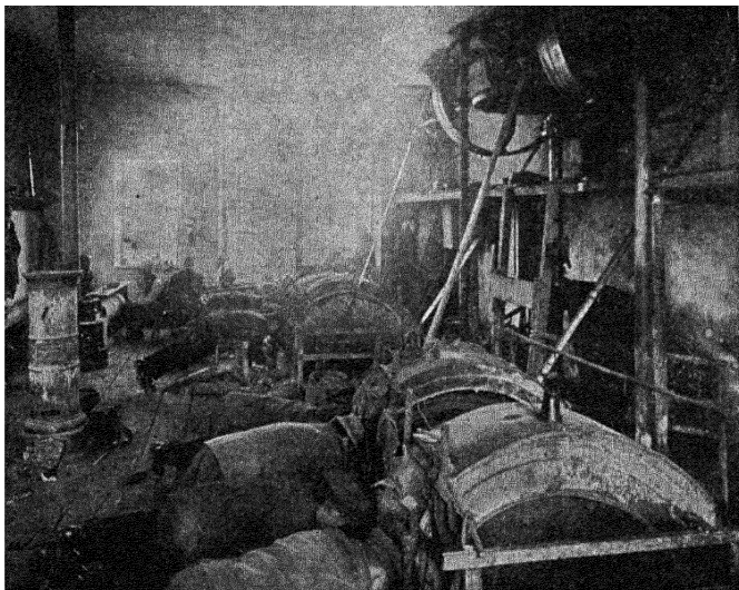
Fig. 158.—Cutting gem stones on large water-driven sandstone wheels at Idar, Germany, where the art has flourished for centuries with but few changes. (Illustration from Gems and Gem Material , Kraus and Slawson, McGraw-Hill Book Company, Inc.)
