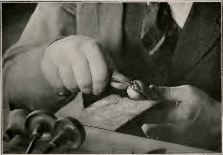
FIGURE 97. Bright cutting top and sides of prongs [159]
