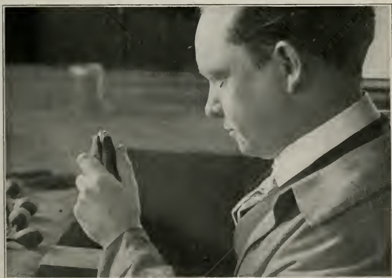
FIGURE 93. Seeing that the stone is level [157]
