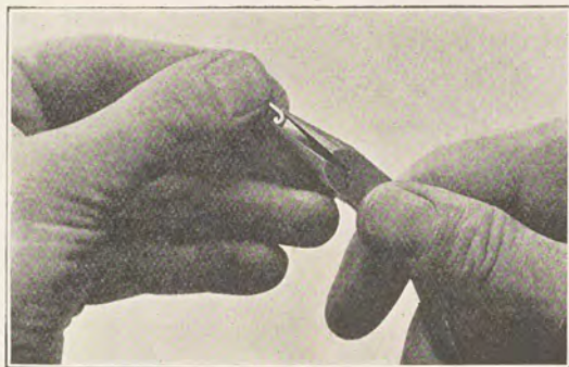
FIG. 54. Curling Flat Wire into a Close Scroll.
